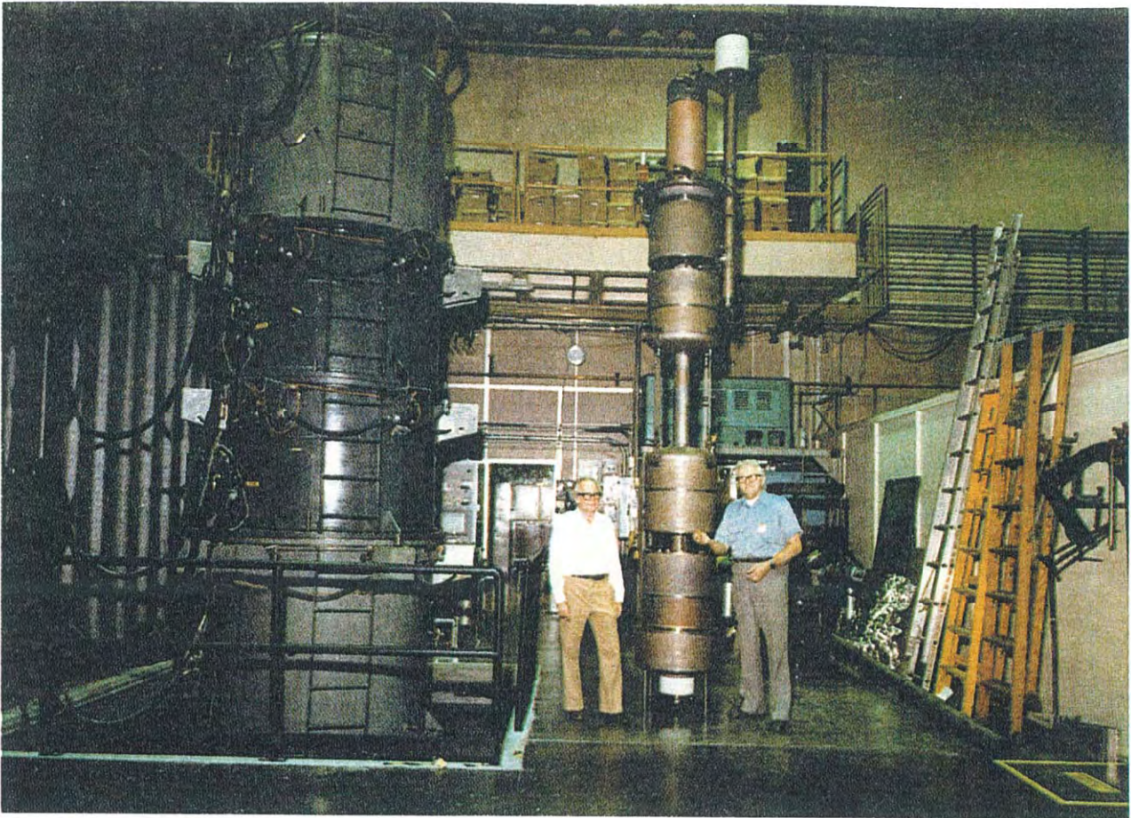
The VHF klystron with magnets removed
