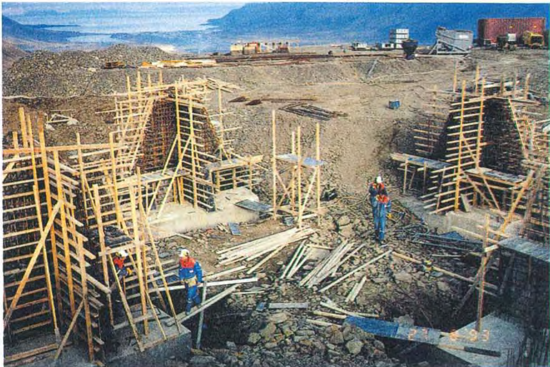
Fig. 7. Construction work on the antenna foundations at the EISCAT Svalbard Radar site on 27 August 1993.
