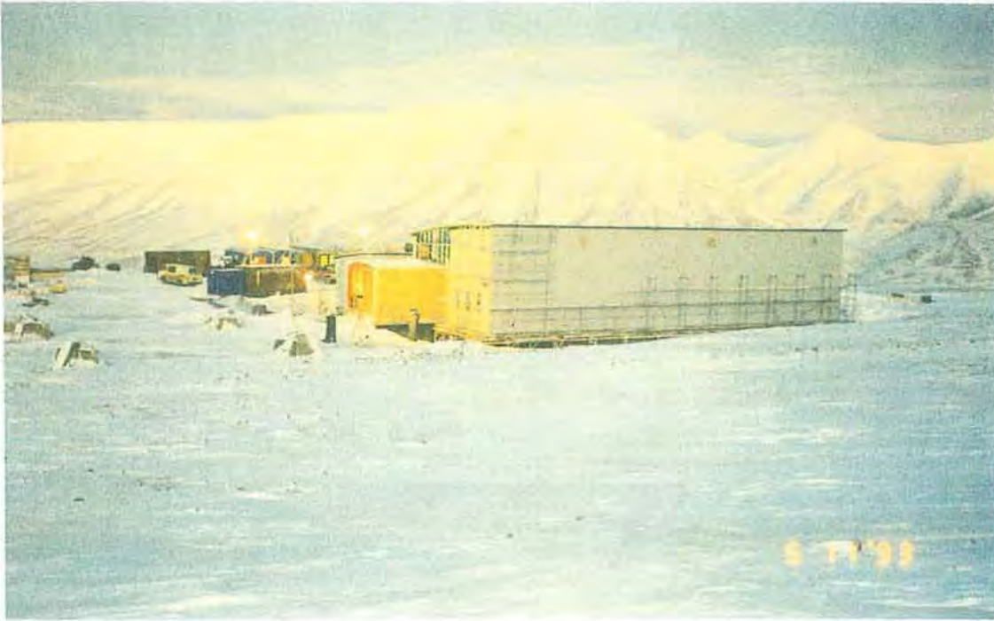
Fig. 8. The EISCAT Svalbard Radar operations building on 5 November 1993. On the left-hand side the four cornerstones of the antenna foundations can be seen.
