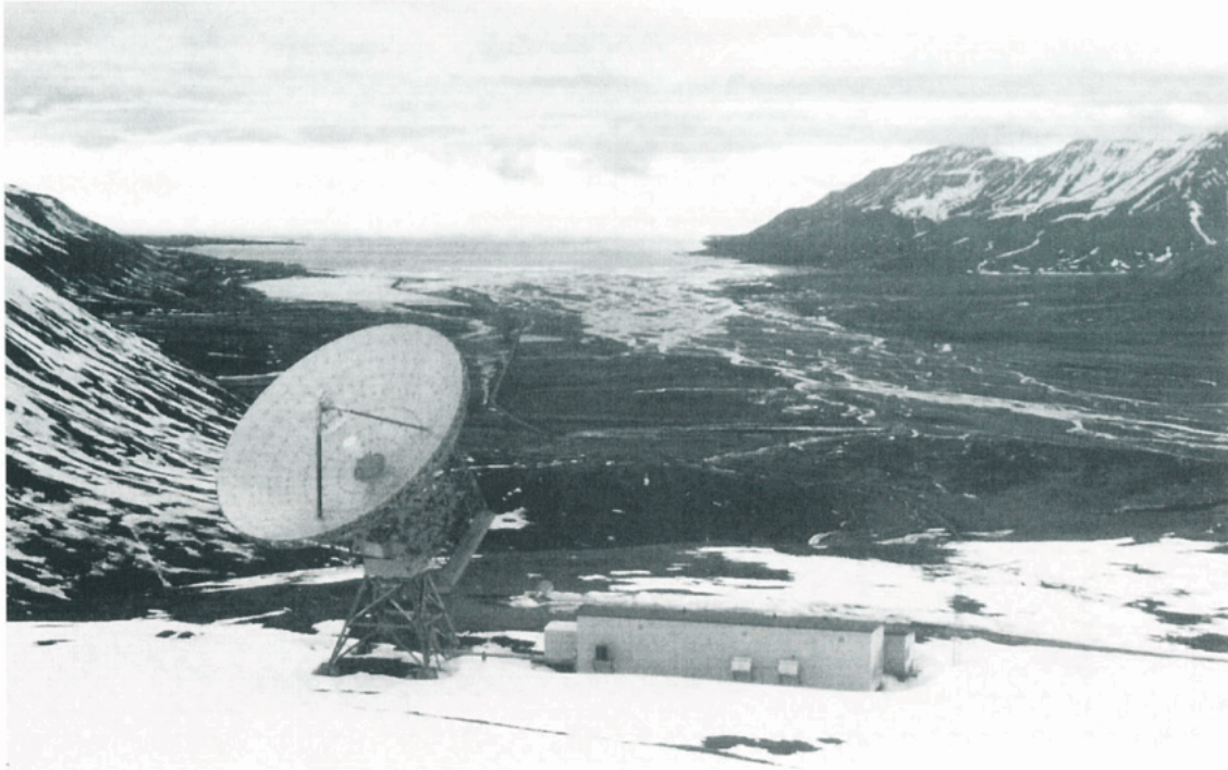
Figure 66: Aerial view of the EISCAT Svalbard radar, looking down the Advent valley toward WNW
