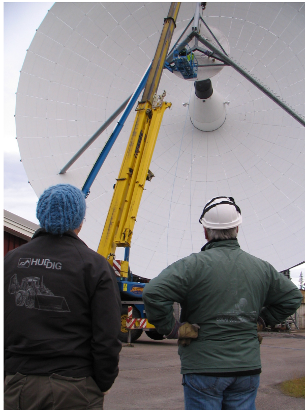
The EISCAT receiver stations in Kiruna and Sodankylä went through a conversion from UHF to VHF during the year. This necessitated some changes of the antenna hardware. (Photo: William Rideout)
